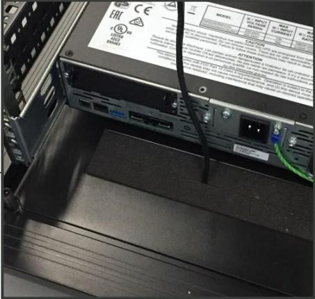
Uncoil the grounding wire, located near the rear bottom of the rack, and connect to the building's electrical ground. Ensure that connections are tightly fastened.
